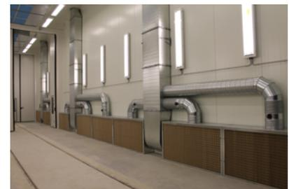
Painting chamber **ventilation** is carried out by explosion-proof low pressure radial fans and has a vertical direction, which implies a top-to-bottom air movement inside the chamber. Such air distribution scheme eliminates the risks from the sideways air movement, which is spraying on the previously painted surfaces. Air velocity in the chamber is sufficient for the timely disposal of hazardous gases from the chamber and meets the EN specified standards.
